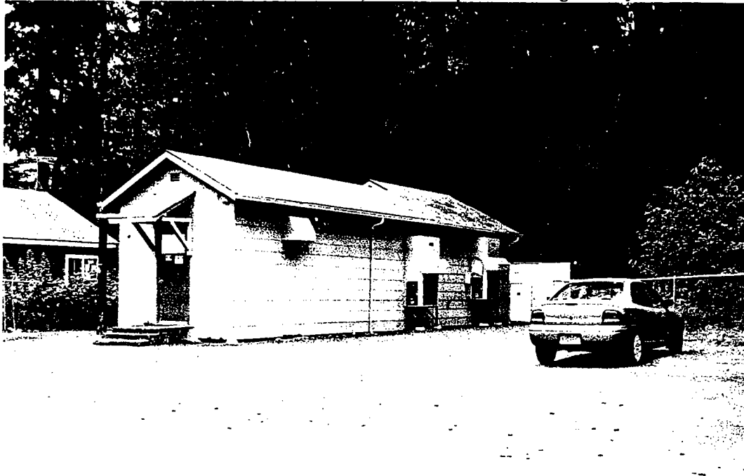
Photograph of the subject property: Qwest Corporation telephone exchange facility.
